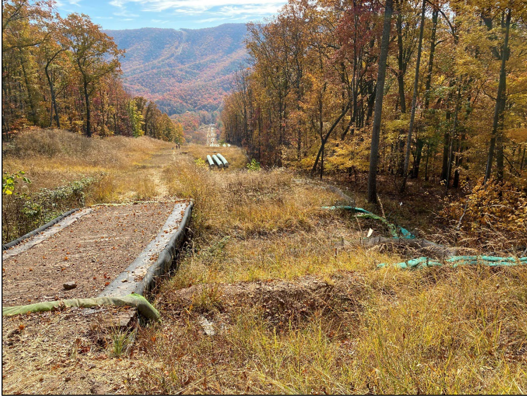
Stream PP22 Crossing on Sinking Creek Mountain (October 2022).
