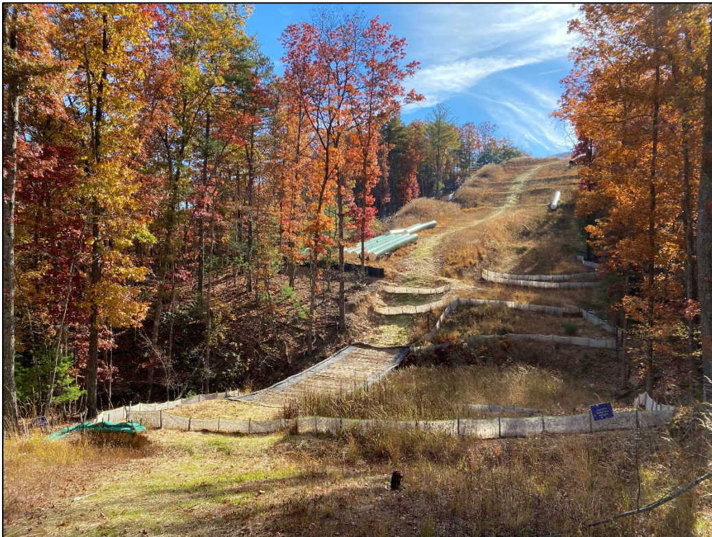
Stream HH18 Crossing on Brush Mountain (October 2022).
