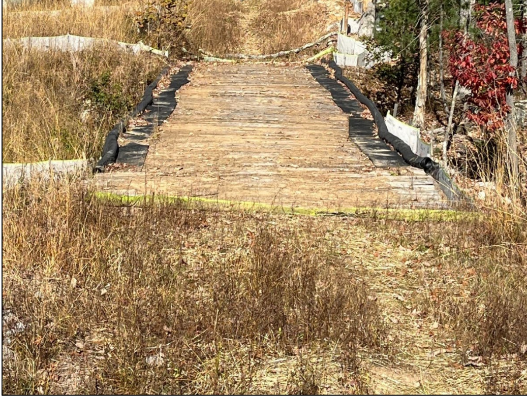
Stream PP20 Crossing on Sinking Creek Mountain (October 2022).
