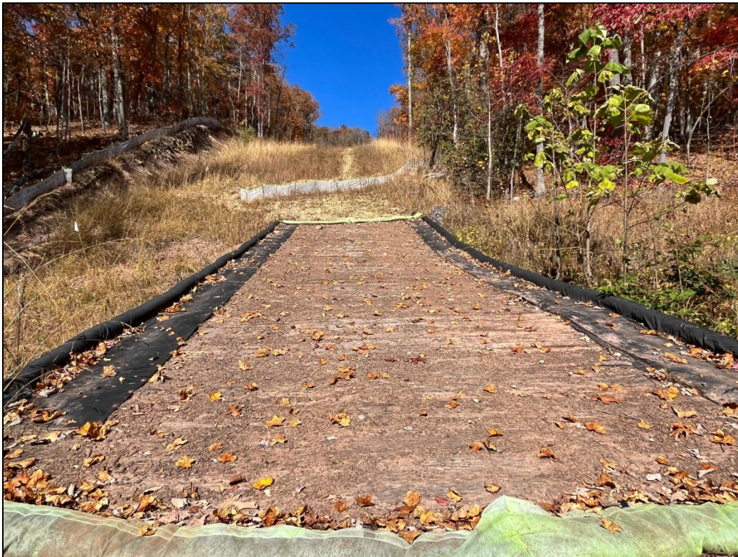
Stream PP21 Crossing on Sinking Creek Mountain (October 2022).
